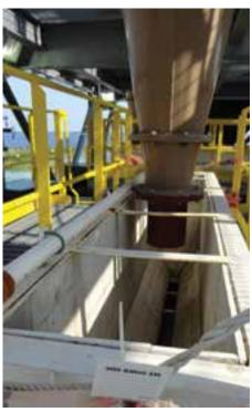
One of many ways to provide feed to the CrossFlow. In this case, cyclone underflow is discharged directly into the ceramic-lined feed box of a 3x3 meter (10x10 ft) CrossFlow Separator.
